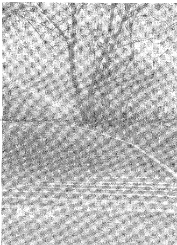
Stepping into the future — pathways are built and the new park begins to take shape.
