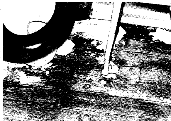
Rotting floorboards in the bathroom of one of the Calders flats. Pic. Martyn Petrie.
